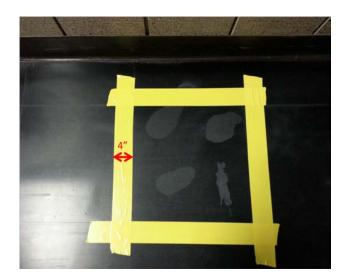
Apply  $3M^{\text{TM}}$  471 Vinyl Tape around the area to be repaired. For floor tiles, take care to align the edges of the tiles with the edge of the tape. The tape should cover the tiles neighboring the area to be repaired. Any area that is being repaired should not be covered by tape. The tape should be at least 4" wide around the repair area to protect adjacent areas.
