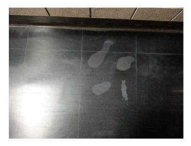
Clean the area to be repaired, taking care to remove all debris and any possible residue that may interfere with coating the floor.
