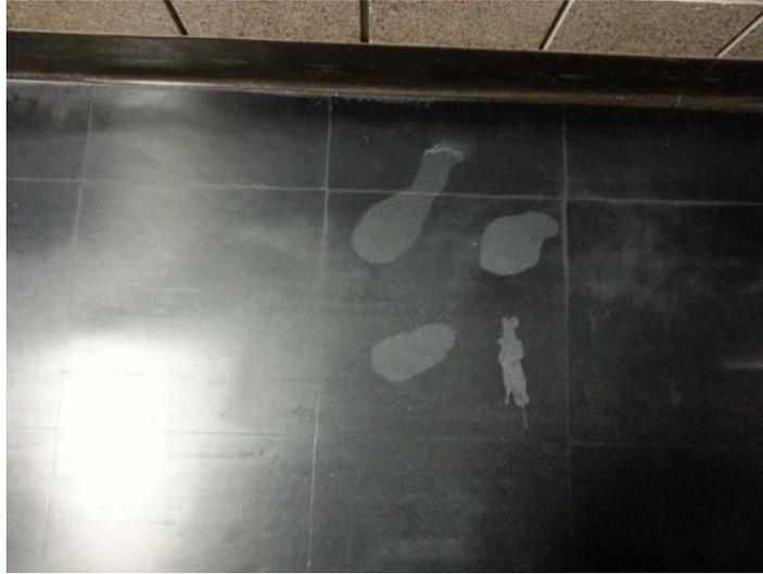
Clean the area to be repaired, taking care to remove all debris and any possible residue that may interfere with coating the floor.
