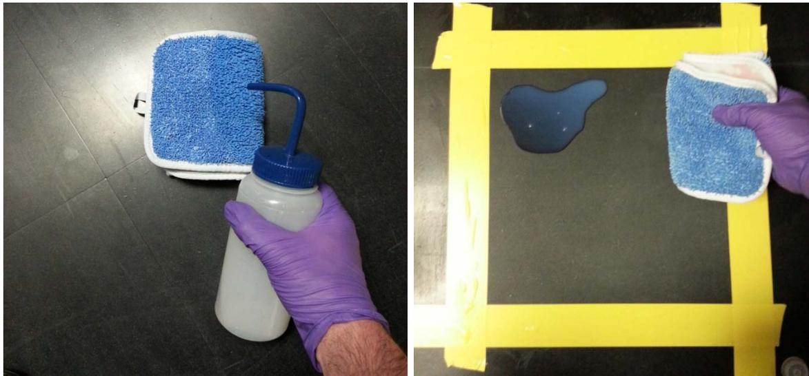
Pre-wet the applicator pad with plain water prior to applying Scotchgard™ Resilient Floor Protector. Wring out the applicator pad so that it is damp, NOT wet. Place a small amount (approx. Silver Dollar sized or 3" diameter circle) of Scotchgard™ Resilient Floor Protector per 12"x12" tile to be repaired (i.e. 4 tiles, 4 small circles).
