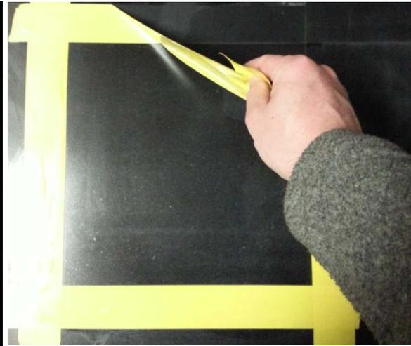
Inspect the repair area for a missed spots, surface integrity and overall condition. If an error was made during the repair process, steps 3-6 can be repeated to ensure a proper repair. After inspection of a successful repair, slowly remove the tape by using constant, consistent motion. Do not clean or autoscrub the repaired area for 24 hours.
