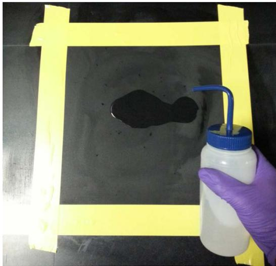
After removing the protector and verifying the repair area is stripped, rinse the area with tap water. Allow the water to cover the repair area for at least 2 minutes. Rinse the repair area a minimum of 2 times. Allow the area to dry before proceeding to the next step.
